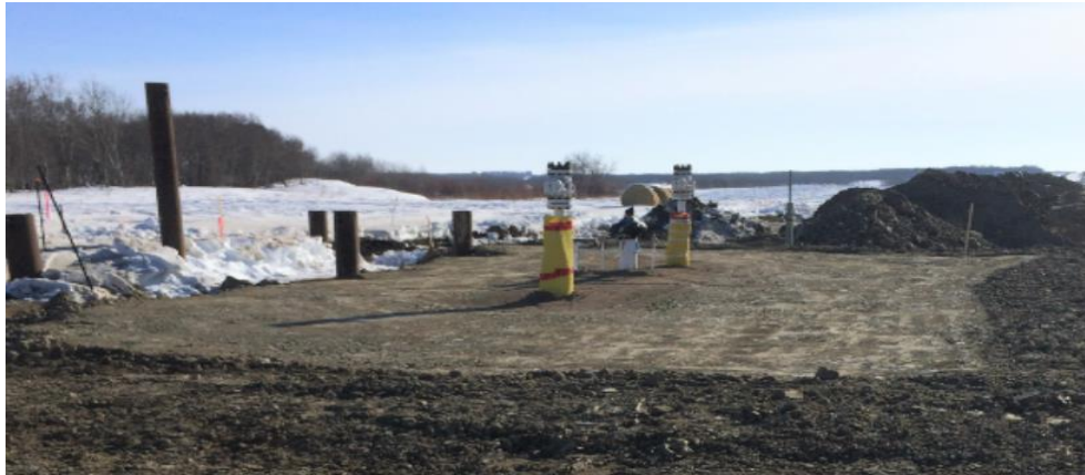
774 + 230 MLBV # 21 Backfill completed
