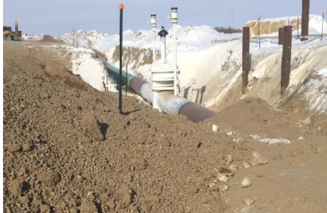
785 + 233 MLBV # 22 Backfilling
