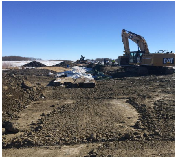
787 + 600 SK WC90 (NFB) Drainage removing ramp
