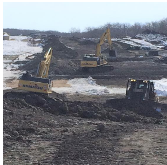
751 + 750 SK WC 87 (NFB) The Little Pipestone removal of the bridge & restoration
