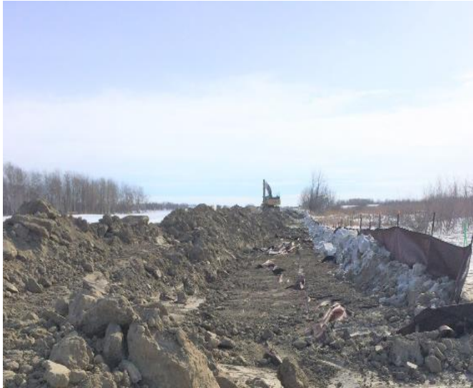
738 + 300 removing ramp at SK 834 Class III
